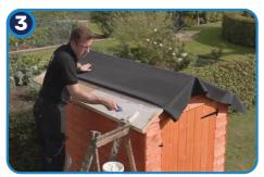
**Apply the adhesive** to the entire roof working 'in stages'. Roll the membrane gradually onto the adhesive whilst wet.
