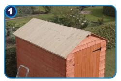
**Remove old roof covering** and nails. Re-board if roof is rotten or roofing felt doesn't come off cleanly.
