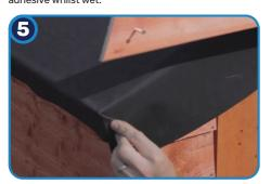
**Reinstall any existing timber** barge boards to help secure the membrane perimeter. Replace if rotten.
