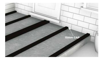
2 A gap of at least 15mm should be left between the ends of Joists and a fixed object such as a wall, and at least 8mm between the ends of Joists at butt joints. These allow for proper drainage and temperature expansion.
